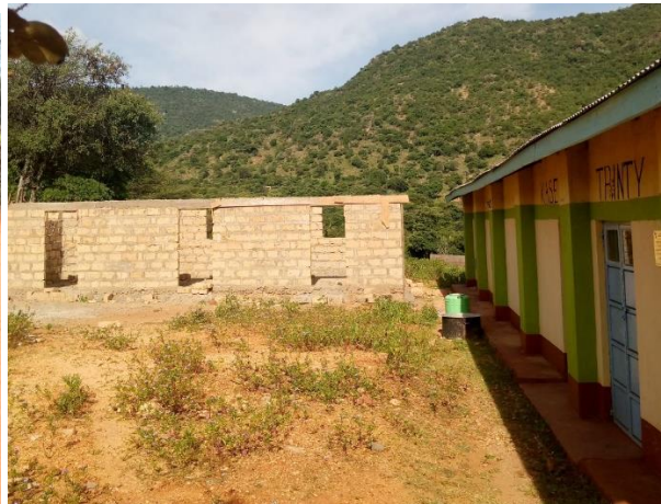
Bible Light construction (left), church building (right)
